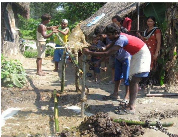
Digging the hole for irrigation in Bhokraha-3, Khoriya tole
